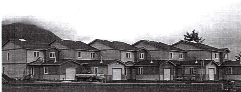
Shuka Hit (Ancestor House), Phase I of the townhouse project
